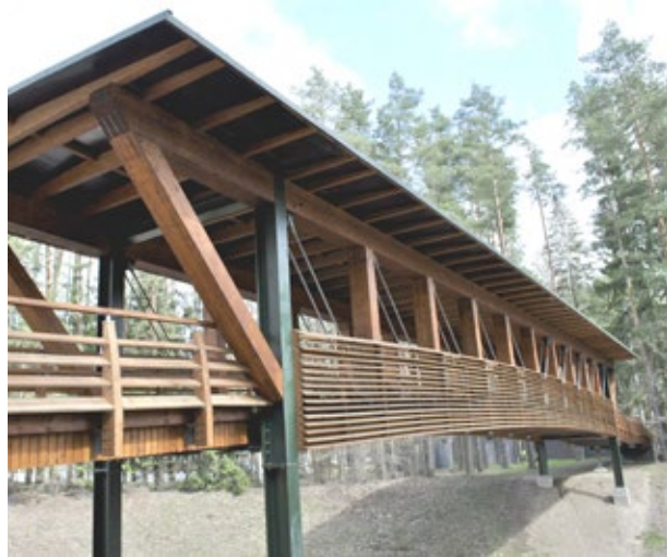
The curved glulam timber beam pedestrian bridge across the road at the entrance to the Tērvete Nature Park was designed, produced, and set up by „JKTK” Ltd.
