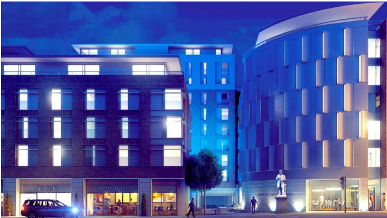
Multi-storey timber building in the city of Liverpool in Great Britain constructed by „Nordic Homes” Ltd
